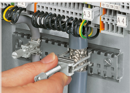
Securing an additional shield clamping saddle.
