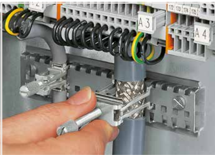
Securing an additional shield clamping saddle.
