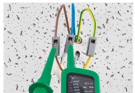
Testing via separate test ports.
