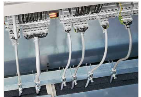
Cable entry in the base of the control cabinet Separate strain relief, movable IP54 bottom plates sealed with sponge rubber (e.g., by Rittal)
