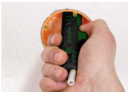
Stripping a cable sheath.
