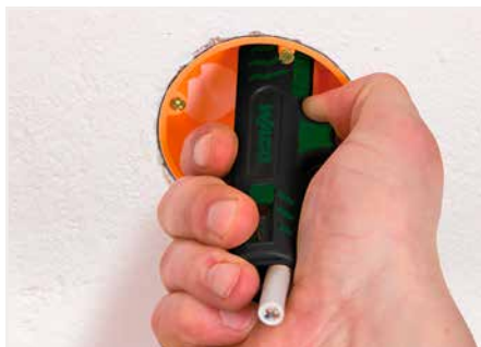
Stripping a cable sheath.
