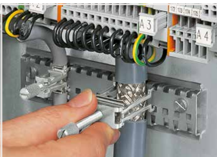
Securing an additional shield clamping saddle.
