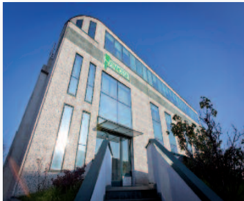
Enerdoor/Finmotor headquarters Milan, Italy
